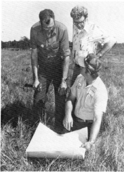
Contractor Wayne Mullenix, kneeling, goes over foundation plans with project superintendent Joe Davis (left) and Georgia Guidestones® builder Joe Fendley prior to actual work being started.
