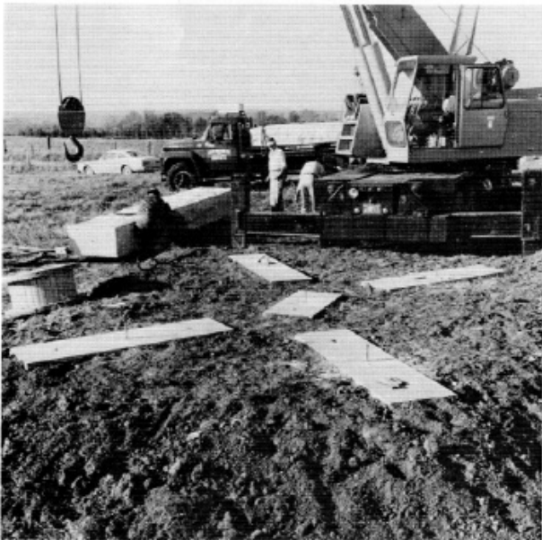
This photo shows the configuration of The Georgia Guidestones® four large outside base slabs, with a central or gnomon stone, arranged like a giant paddlewheel with the outer stones oriented to the limits of the migration of the moon during a year. The center stone is marked and holes drilled in it so that the sun rays mark the time of day and the seasons of the year. Also, the North Star is always visible through a special slot from the South to the North side of the center stone. An astronomer was employed to accurately achieve this placement of the stones.
