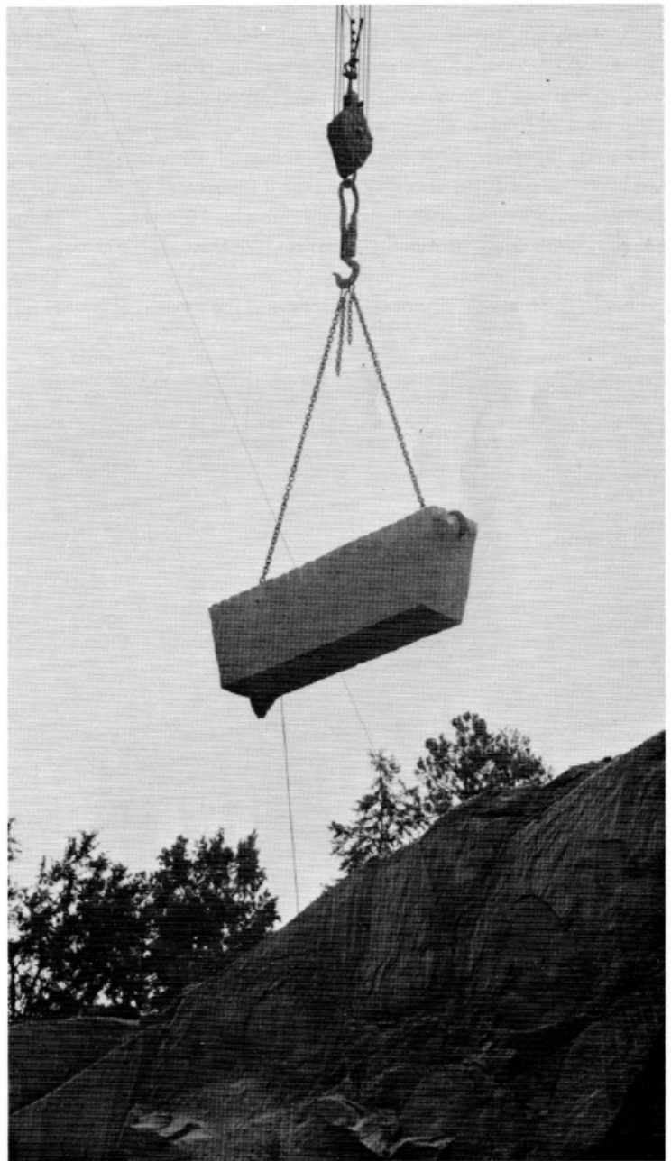
Once the massive pieces of stone were freed from the ledge mass, derricks gingerly lifted them to the rim of the quarry as shown above. Quarrymen were especially wary in this phase, since the derricks normally don't lift such extreme weights.
