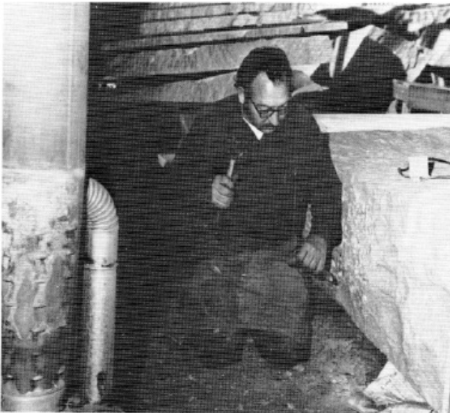
Horace Bradford, one of the two master stonecutters assigned to The Georgia Guidestones® project, is shown smoothing the sides of the center stone.
