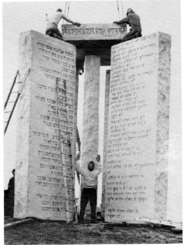
During the waning twilight of March 12, 1960 the final section, the large capstone, was set into place to complete construction of The Georgia Guidestones . Joe Fendley, builder, is shown directing placement of the capstone. All that remained to be done was steam-cleaning the stone for the March 22nd dedication.
