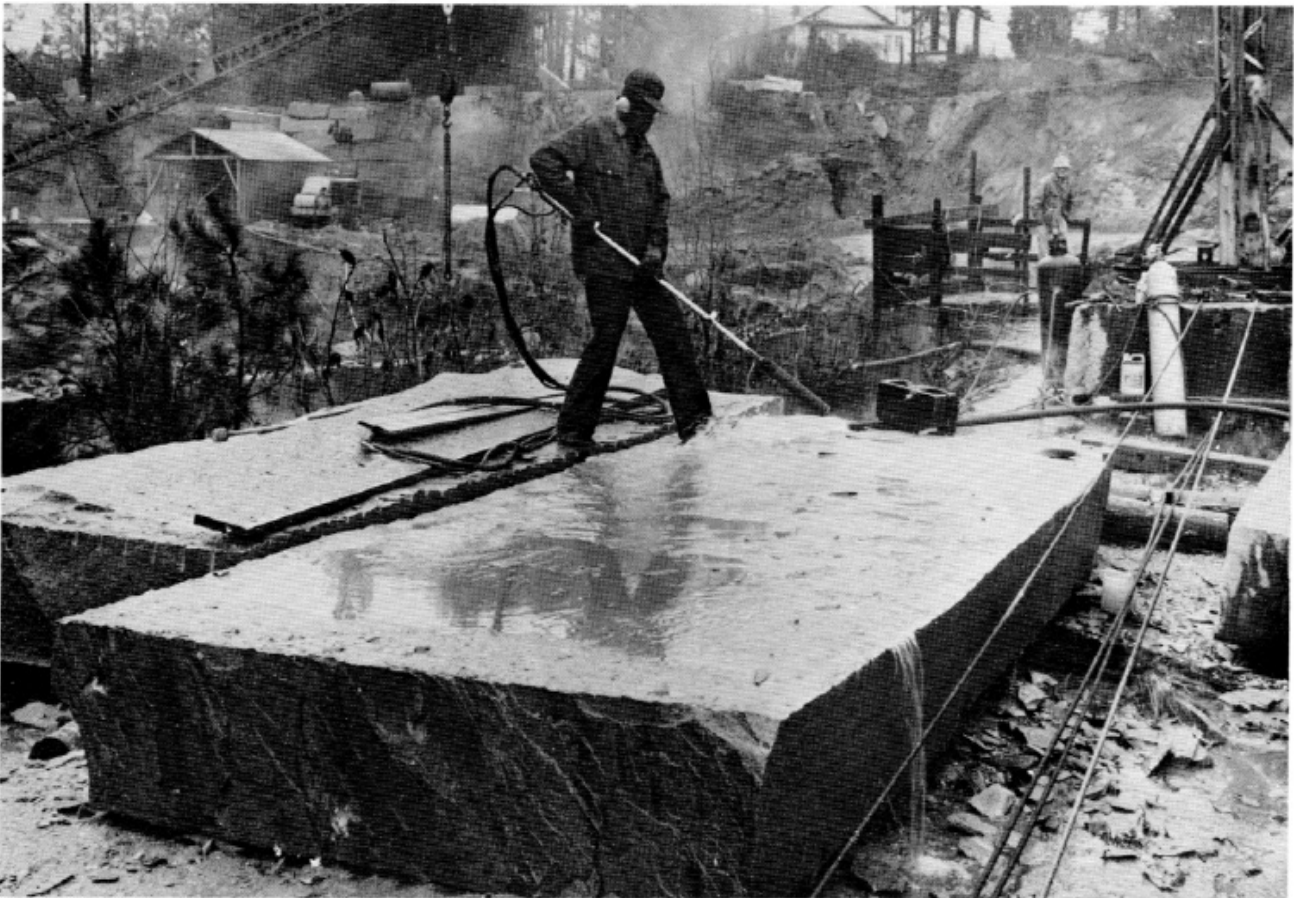
A special "burner" was developed by the C.S. Peck Company to clean and size the large blocks of Pyramid Blue granite which were used for The Georgia Guidestones® project. Shown working on one of The Georgia Guidestones® granite slabs is Henry Smith, Jr. of the Pyramid Quarry crew.
