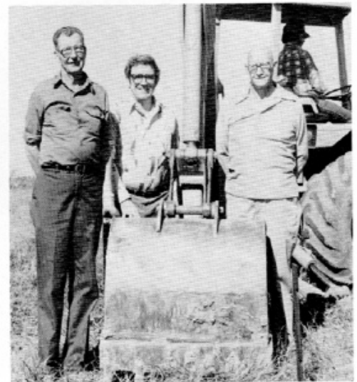
(l-r) Project superintendent Joe B. Davis, builder Joe H. Fendley, Sr., and foundation builder W.A. "Willie" Edwards pause during the early days of construction to pose for the camera.
